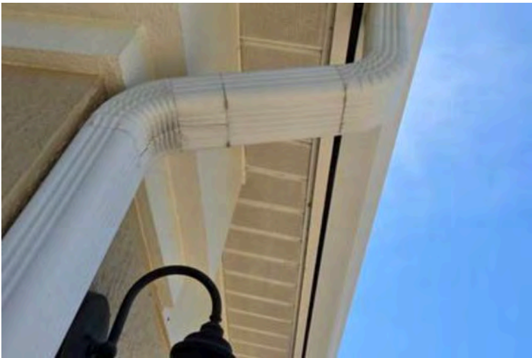
Adequate intake ventilation: perforated soffits
