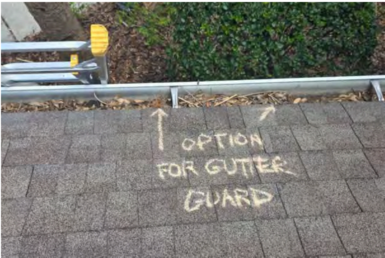
Remove and replace gutter and downspout included. We will include an option for gutter guards, also, to prevent build-up in gutters as displayed.
