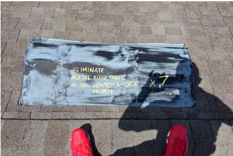
Eliminate 7pc "off-ridge" vents. These historically allow wind driven rain into the attic. The new ridge vent will provide a safe and proper attic exhaust system.
