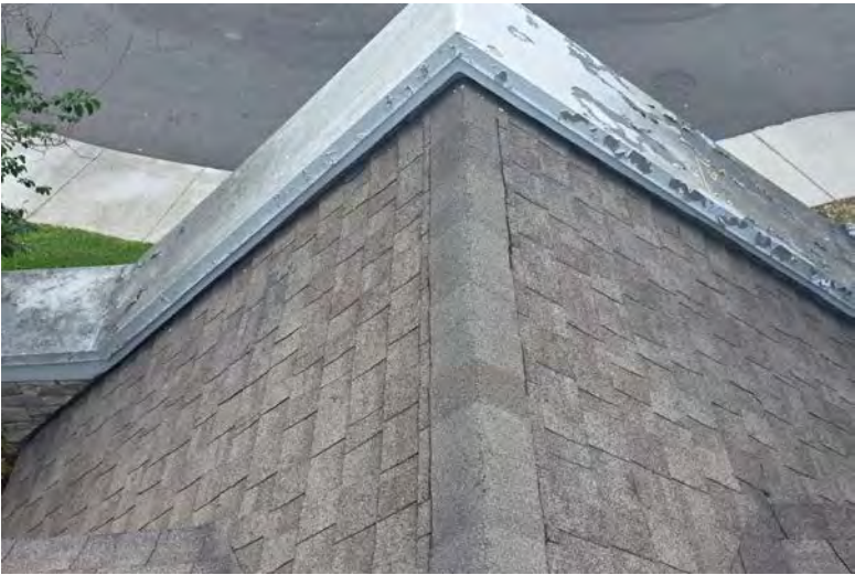
Remove and replace wall coping #2
