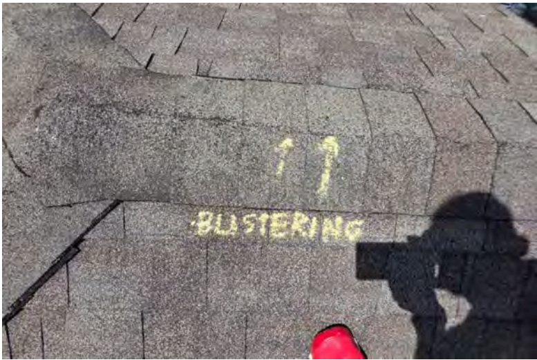
Due to inadequate exhaust ventilation expelling hot air from the attic, existing shingles are blistering, or "cooking from the inside out." We will vent all ridges with a new ridge vent system.
