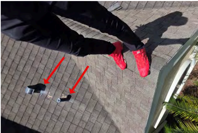
Remove & replace all penetration flashings and exhaust vents
