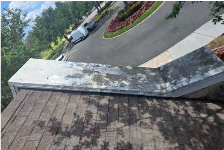
Remove and replace wall coping included, using 26ga metal coping. Color TBD.
